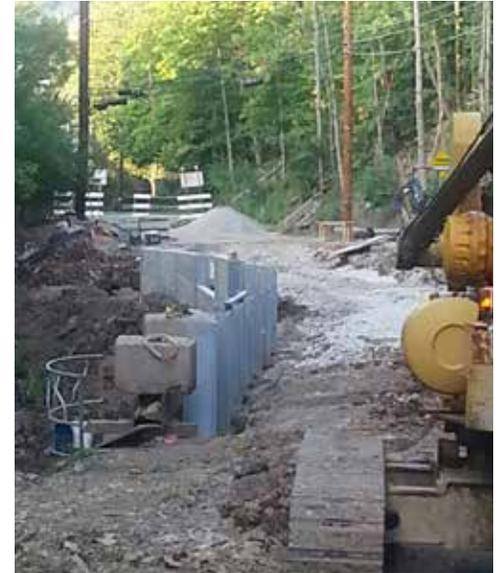
Aug 23<sup>rd</sup> - Installed soldier piles for the retaining wall
