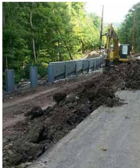
Sept 2<sup>nd</sup> - Concrete lagging installed for the retaining wall
