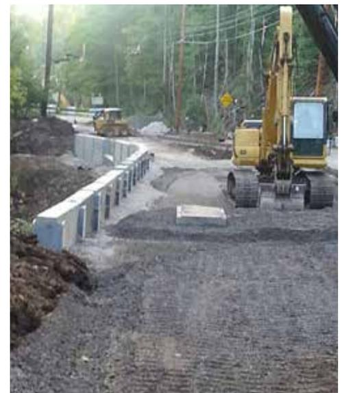
Sept 15<sup>th</sup> - Backfilling and grading the road- preparing for paving
